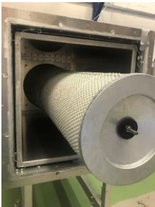
Upstream view of filter pair
